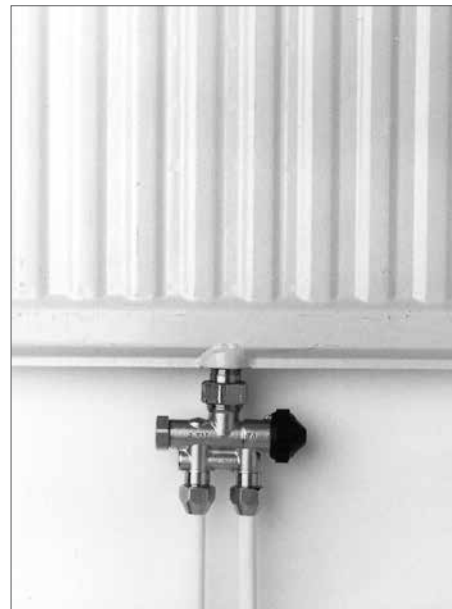
1-strengsventil, undermonteret
