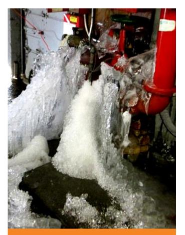
In this example, after a power supply breakage, the valve remained at its closed position not enabling a minimum flow to prevent pipe freezing. This led to repair costs 242 k€ and a shutdown of the HVAC system.
