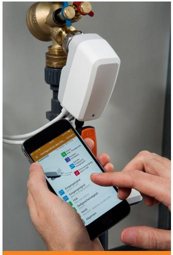
The **TA-Slider** actuator is fully configurable via the **HyTune app**
